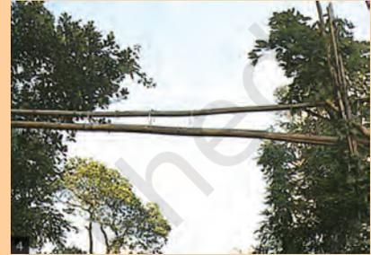
*Picture 2 and 3: The channel sections, made of bamboo, divert water to the plant site where it is distributed into branches, again made and laid out with different forms of bamboo pipes. The flow of water into the pipes is controlled by manipulating the pipe positions.*
